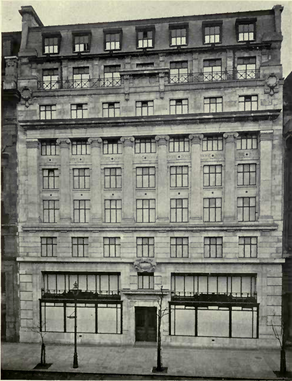
PRINCE'S HOUSE, KINGSWAY.
